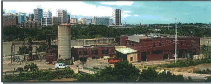
Figure 8: Vacant Land and the dilapidated Federal Paper Mill
